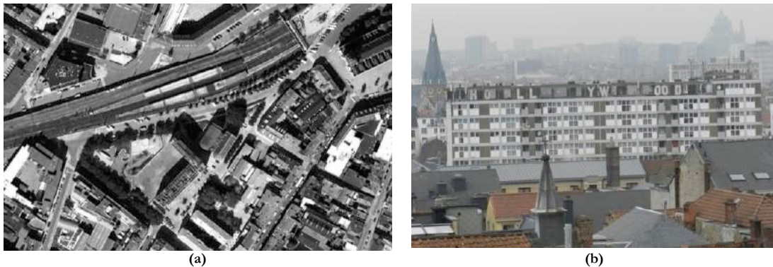
Figure 4.2: Air photo of the site, source: Google Earth (a); View on the Brigittinnen building from the Justice Court of Brussels (b)
