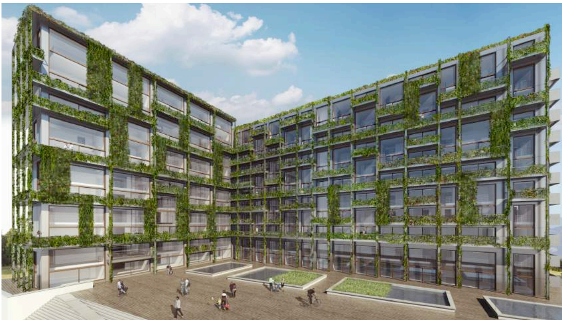
Figure 4.19: New "double" west façade: combination of technosphere (first façade) and biosphere (second façade)
